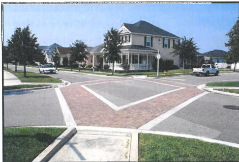
Crosswalk with colored and textured pavement. www.pedbikeimages.org/ (Dan Burden)
